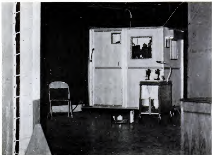
Special Holmes 16-mm. projector , in portable soundproof booth, is used by N.B.C. to create movie backgrounds. Projector, designed
